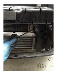
12. Remove crash bar 3x13mm bolts + 2x T30 bolts each side.
