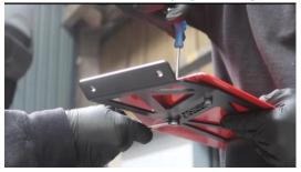
4. Carefully mark out drill holes using templates provided.
