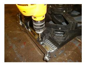
2. Once you have drilled the holes into the surround, hook it back onto the radiator and secure with bolts provided.
